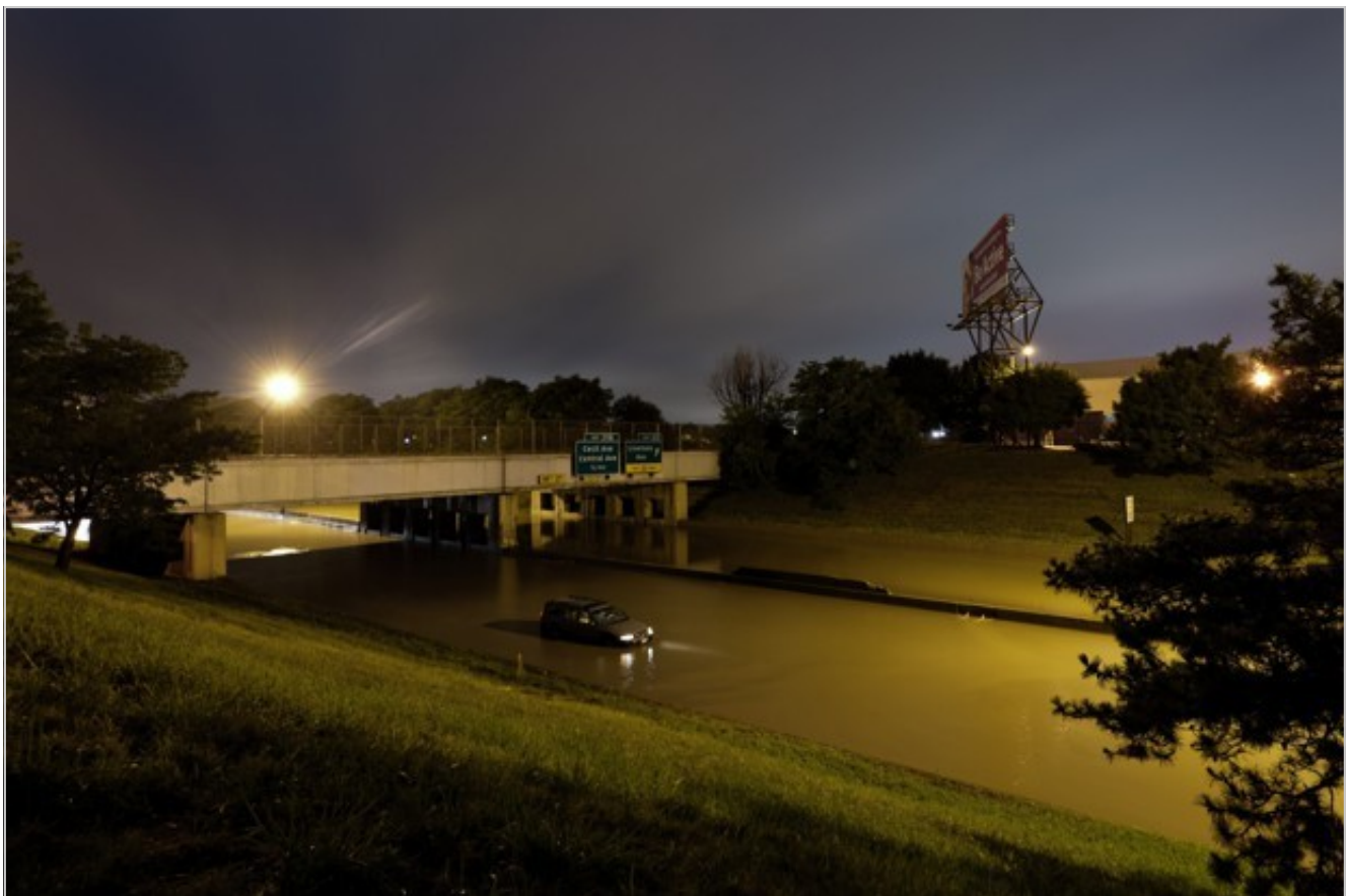
"Edsel Ford River, Supermoon Sewer Slam, 2014" (Scott Hocking)
